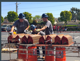
Figure 5. Steel Bridge Loading
